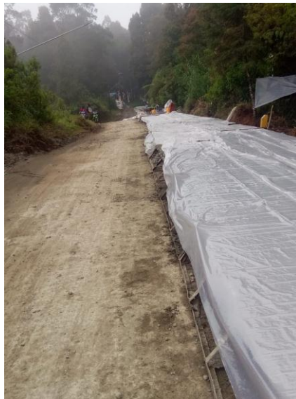
Gambar 8.4 Perawatan Beton
